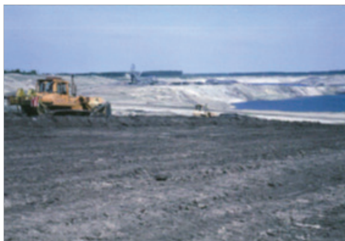
Fig. 2: Preparation of final slopes in Lubstów open-pit (KWB Konin).
