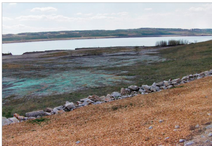
Fig. 14: Shore line with anti-abrasive system (Photo: P. Valvoda, 04/2013).
